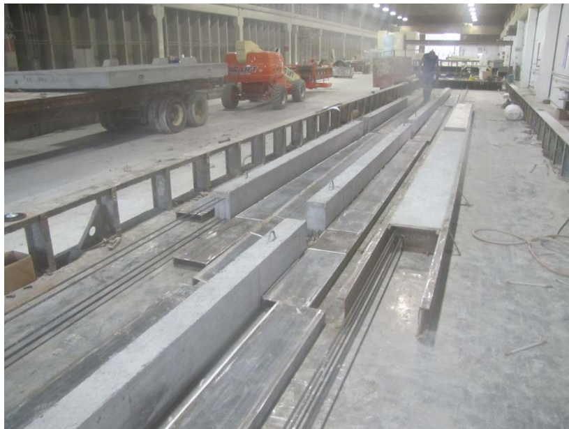
Figure 4.9 – Beams After Form Removal and Before Instrumentation
