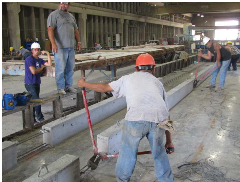
Figure 4.10 – Bolt Cutting Strands at Release
