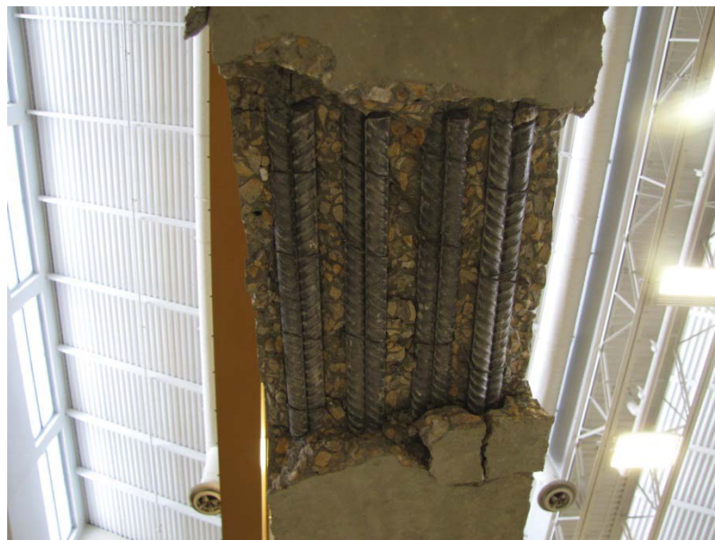
Figure 5.14 – Bottom of splice region of C10-58LTB with splice revealed
