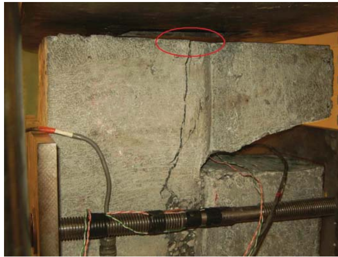
(a) Cracking and Downward Movement of End Corbel
