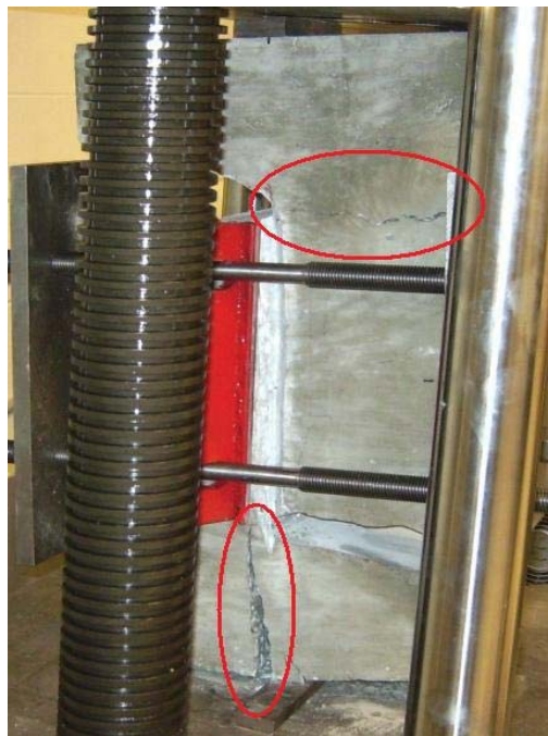
(b) Cracking and Rotation of End Corbel
