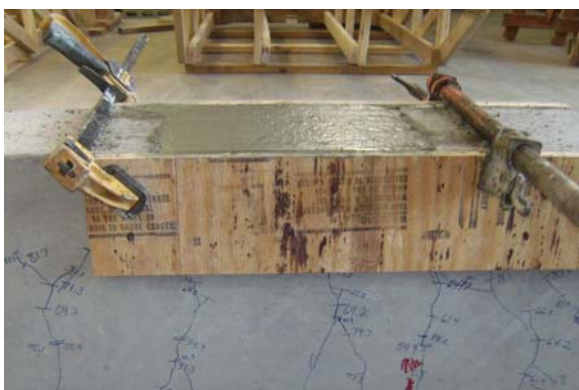
(d) "Scrub coat" and grout placed, finished (e) Cured under burlap and plastic sheeting
