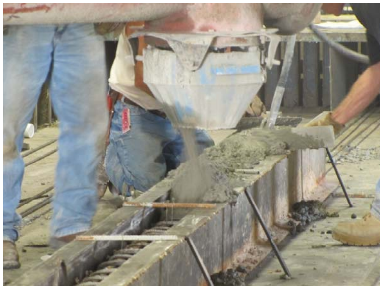
Figure 7.8 – Coreslab Structures, Inc. Crew Places, Consolidates, and Finishes Concrete for Beams
