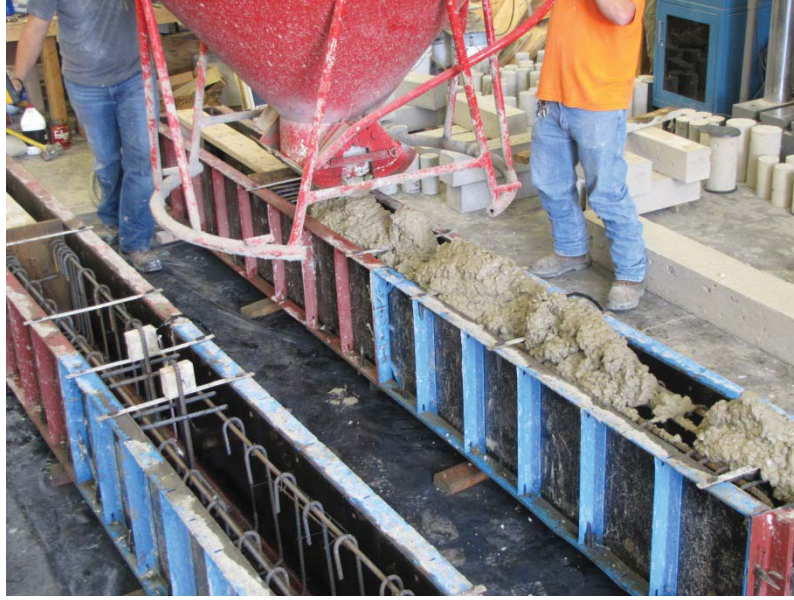
Figure 4.13 – Placement of concrete into beam forms
