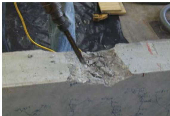
(a) Damaged area chiseled (b) Hammer drill used to chisel deep into the member
