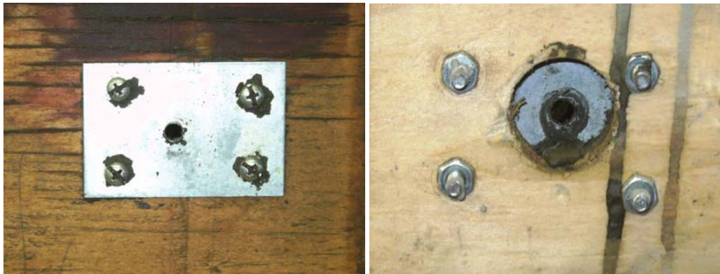
(a) Inside Forms, Metal Sheet Attached with a Hole Drilled
