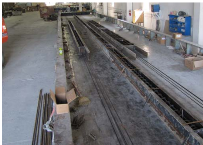
(d) Full prestressing bed with bond and shear beams in place
