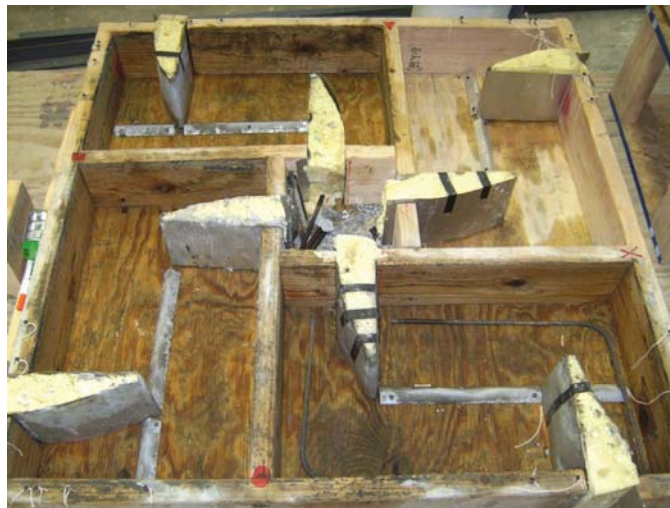
Figure 6.16 – Complete Initial Formwork, Up To Four Specimen Cast at a Time
