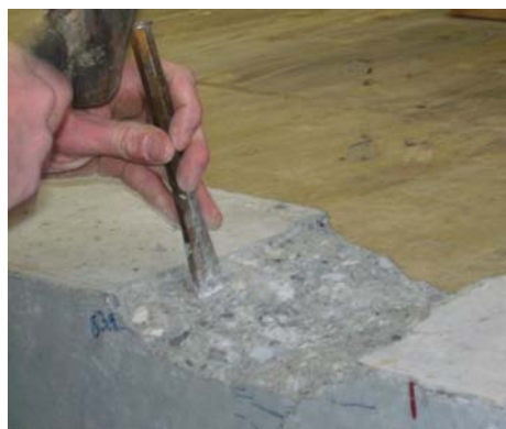
(a) Damaged area chiseled (b) Hammer drill used to chisel deep into the member
