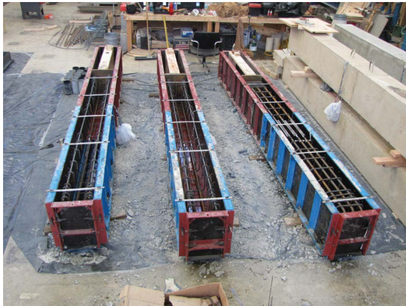
Figure 4.11 – Reinforcing bar cages in beam forms
