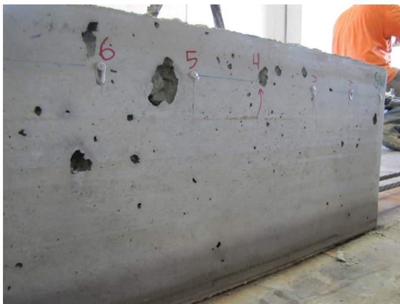
Figure 4.12 – Honeycombing Preventing DEMEC Placement at Point 4 on C10-4-1_SW
