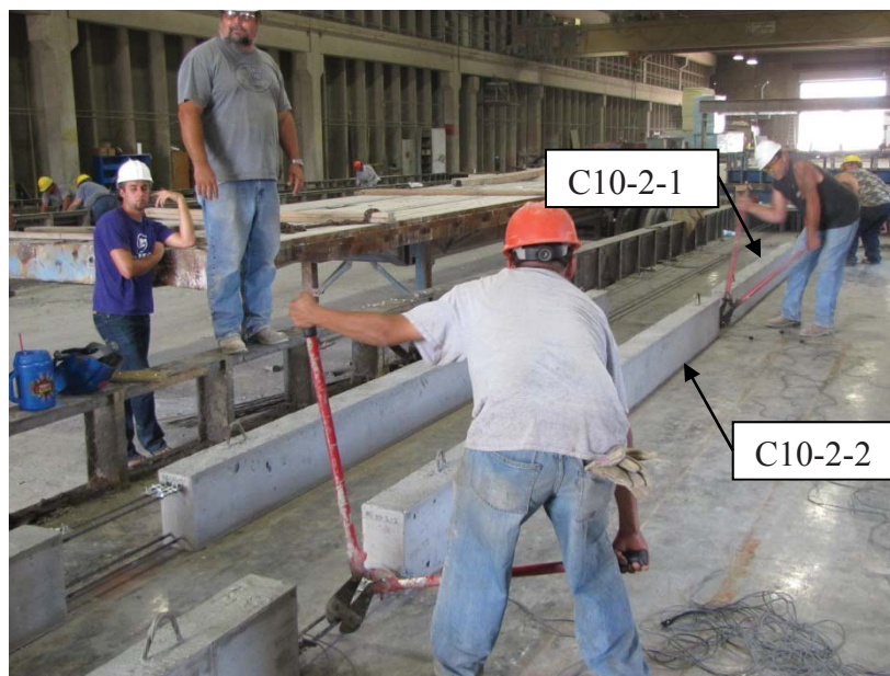
Figure 5.14 – Release of C10-2 Beams
