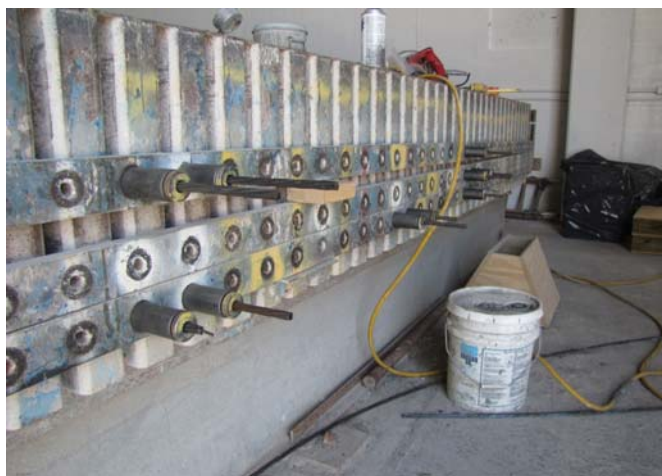
(a) "Dead end" steel tendons anchored into position
