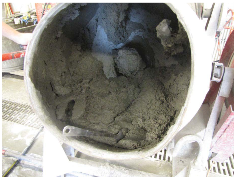
Figure 3.7 – Mortar Mix in Drum Mixer
