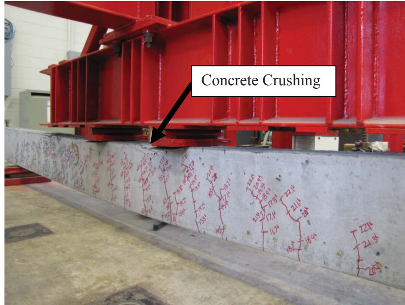
Figure F.19 – C10-2-1_73 at Failure
